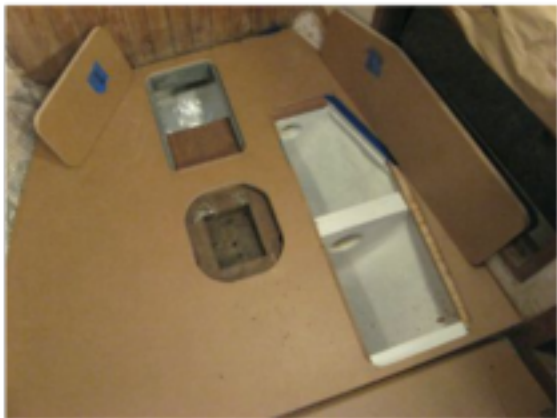
New Floor Panels
